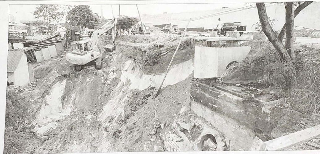
AN excavator proceeds with the preparatory work for the expansion of Nyerere Road near Chang'ombe flyover in Dar es Salaam as captured yesterday. (Photo by Mohamed Mamba)
